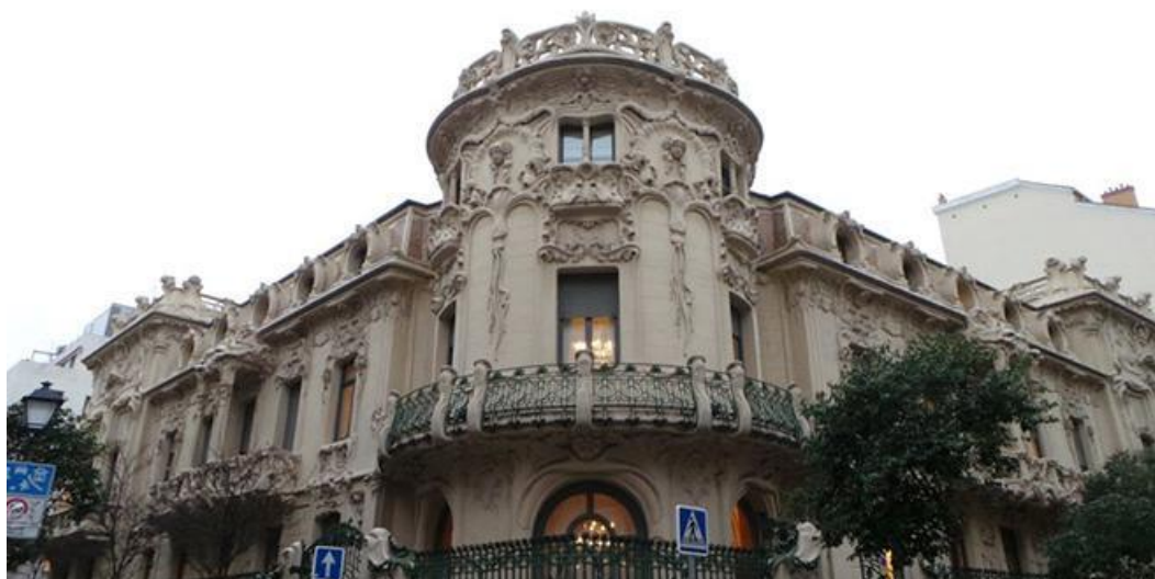
FIGURE 6. SGAE HEADQUARTERS, MADRID (SPAIN)
